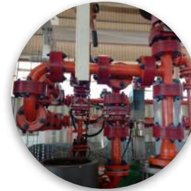
Piping Modification Works
