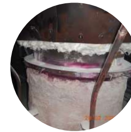
Stiffener Ring Rectification Works
