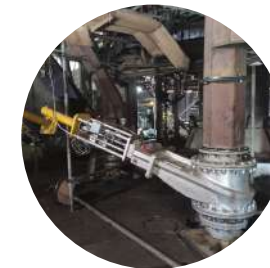
Feed Chutes & Hydraulic Knife Gate Installation
