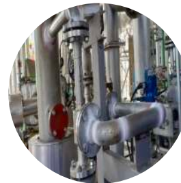
Piping & Equipment Shutdown & Turnaround Works
