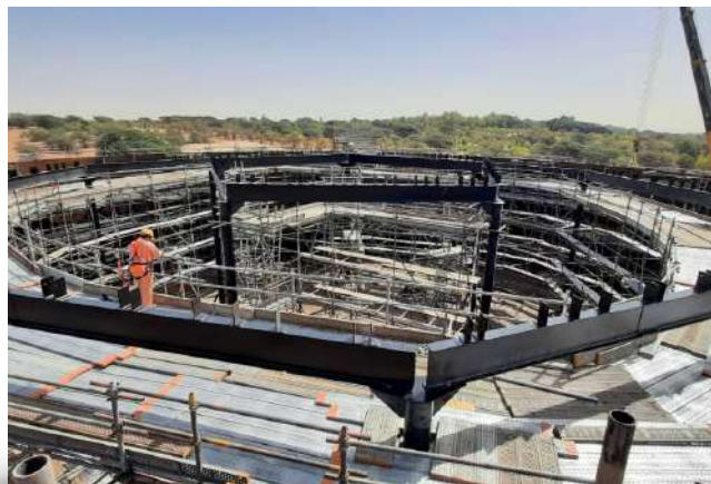
Larsen & Toubro Storage Tank Erection Project, Abu Dhabi, UAE
