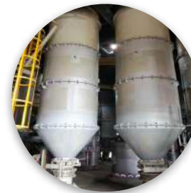
Furnace Feed Chute Cladding & Structure Strengthening Works
