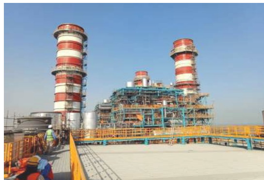
Jebel Ali Power Plant, Dubai, UAE
