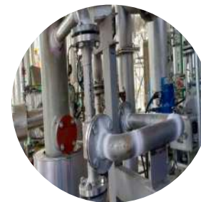
Piping & Equipment Shutdown & Turnaround Works
