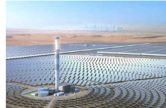
Al Maktoum Solar Park, Dubai, UAE
