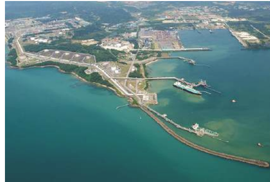
PETRONAS BAGSF2, Bintulu, Sarawak
