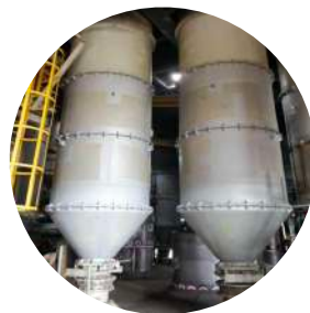
Furnace Feed Chute Cladding & Structure Strengthening Works
