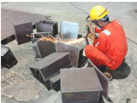
Fabrication Works (Cutting, Fit-Up & Welding)
