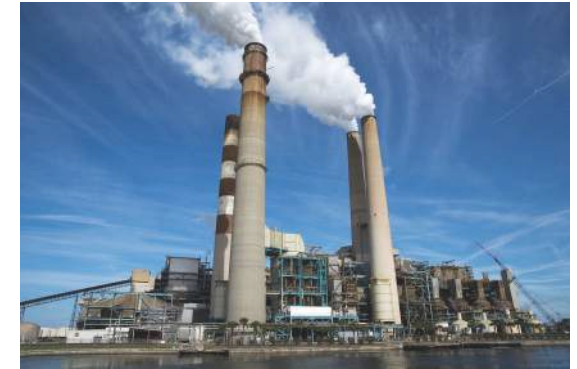
Hamriyah Power Plant, Sharjah, UAE
