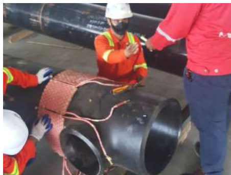
Post Weld Heat Treatment (PWHT)
