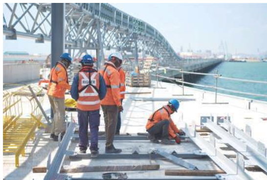
Petronas RAPID Project, Pengerang, Johor
