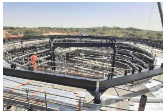
Larsen & Toubro Tank Erection, Abu Dhabi, UAE
