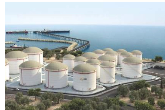
ATB Oil Terminal, Tanjung Bin, Johor
