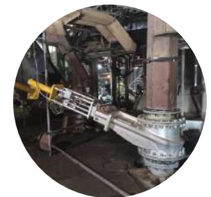
Feed Chutes & Hydraulic Knife Gate Installation
