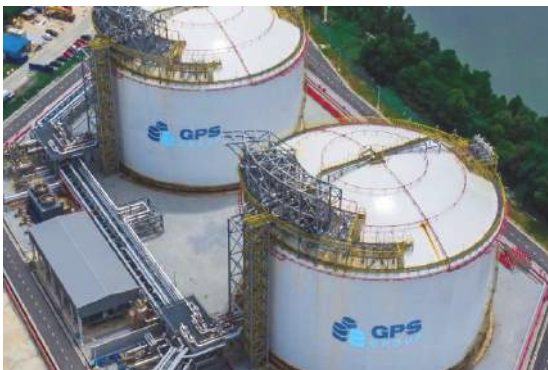
GPS LPG Terminal, Port Klang, Selangor
