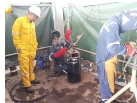
Welder Qualification Test (WQT)
