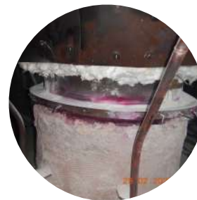
Stiffener Ring Rectification Works
