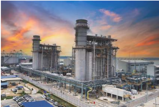
GE Power SIPP Plant, Johor
