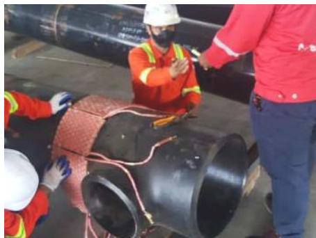
Post Weld Heat Treatment (PWHT)
