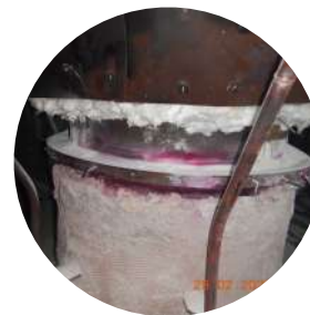
Stiffener Ring Rectification Works
