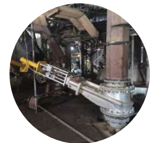
Feed Chutes & Hydraulic Knife Gate Installation
